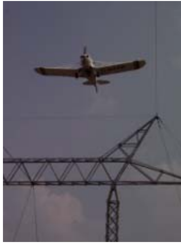
Fig. 1. Aerial power line inspection illustration (from News Releases).
